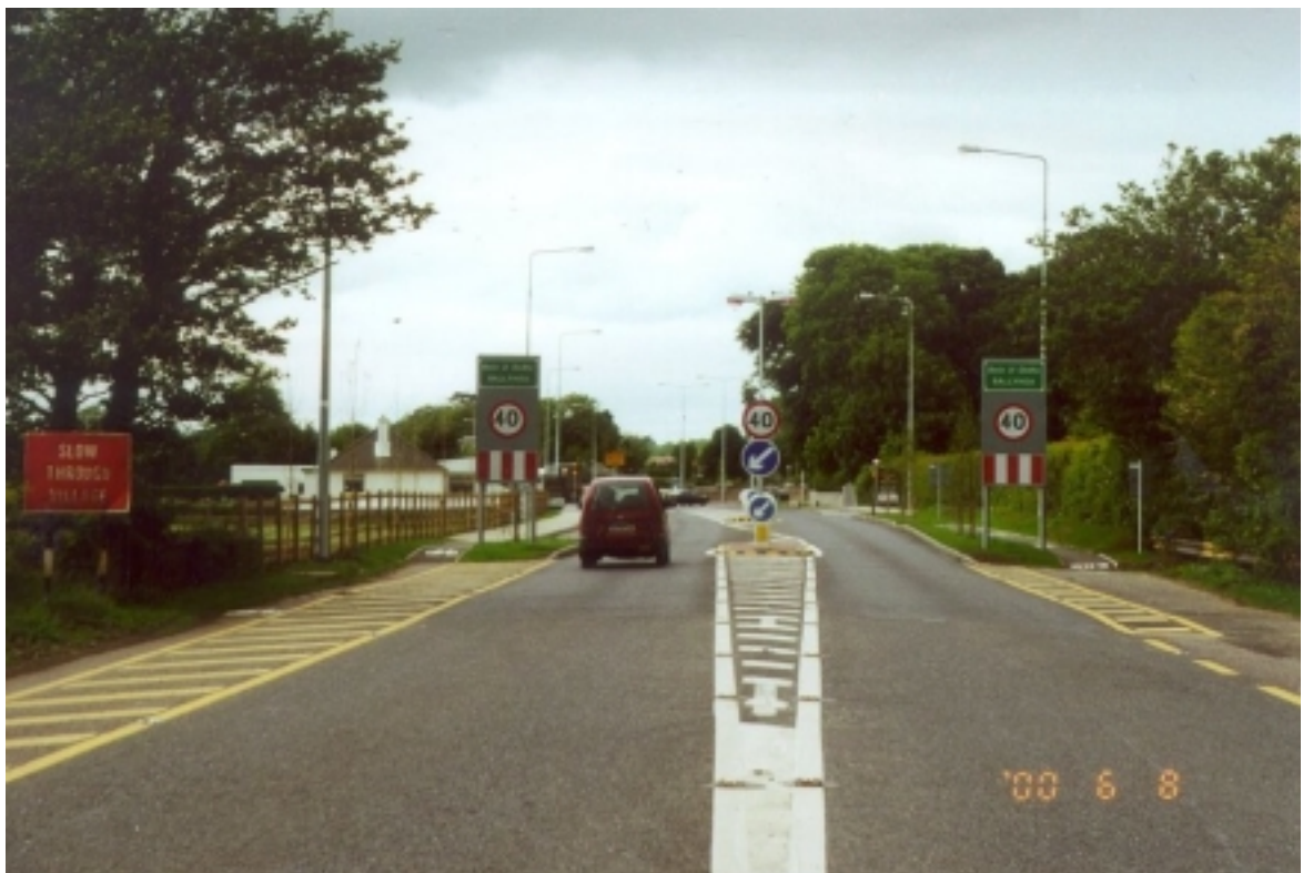
Photo 5: N20 Ballyhea, Co. Cork – South Approach ‘after’
