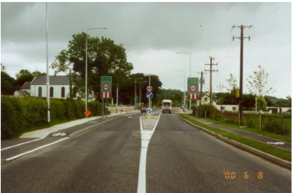
Photo 3: N20 Ballyhea, Co. Cork – North Approach ‘after’
