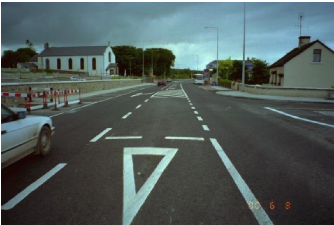
Photo 7: N20 Ballyhea, Co. Cork – Staggered Junction ‘after’
