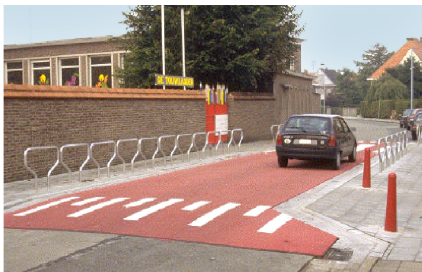
Figura 9 - Una piattaforma lunga davanti ad una scuola (fonte: European Commission, 1998, Adonis - Analysis and Development of New Insight into Substitution of Short Car Trips by Cycling and Walking)
